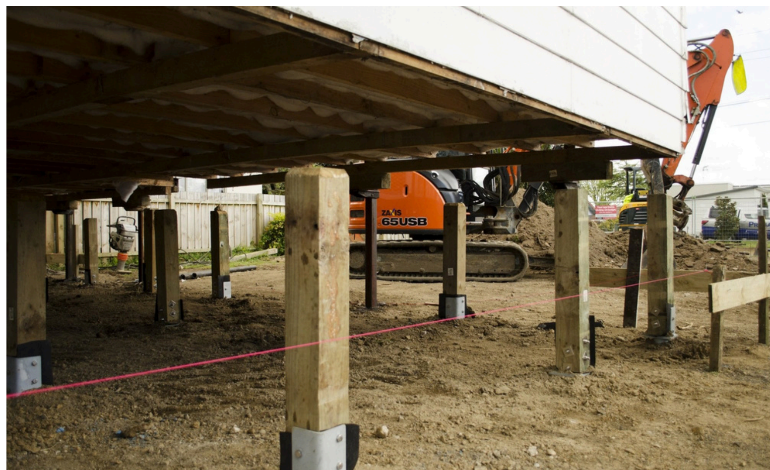
— Timber post connection for relocatable buildings.
