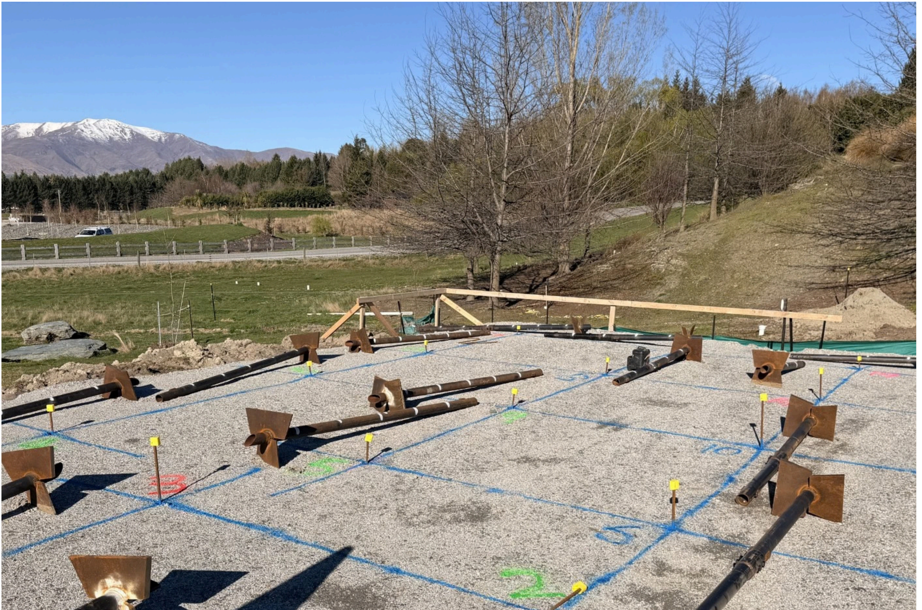
— Blade Piles set out and ready for installation.
