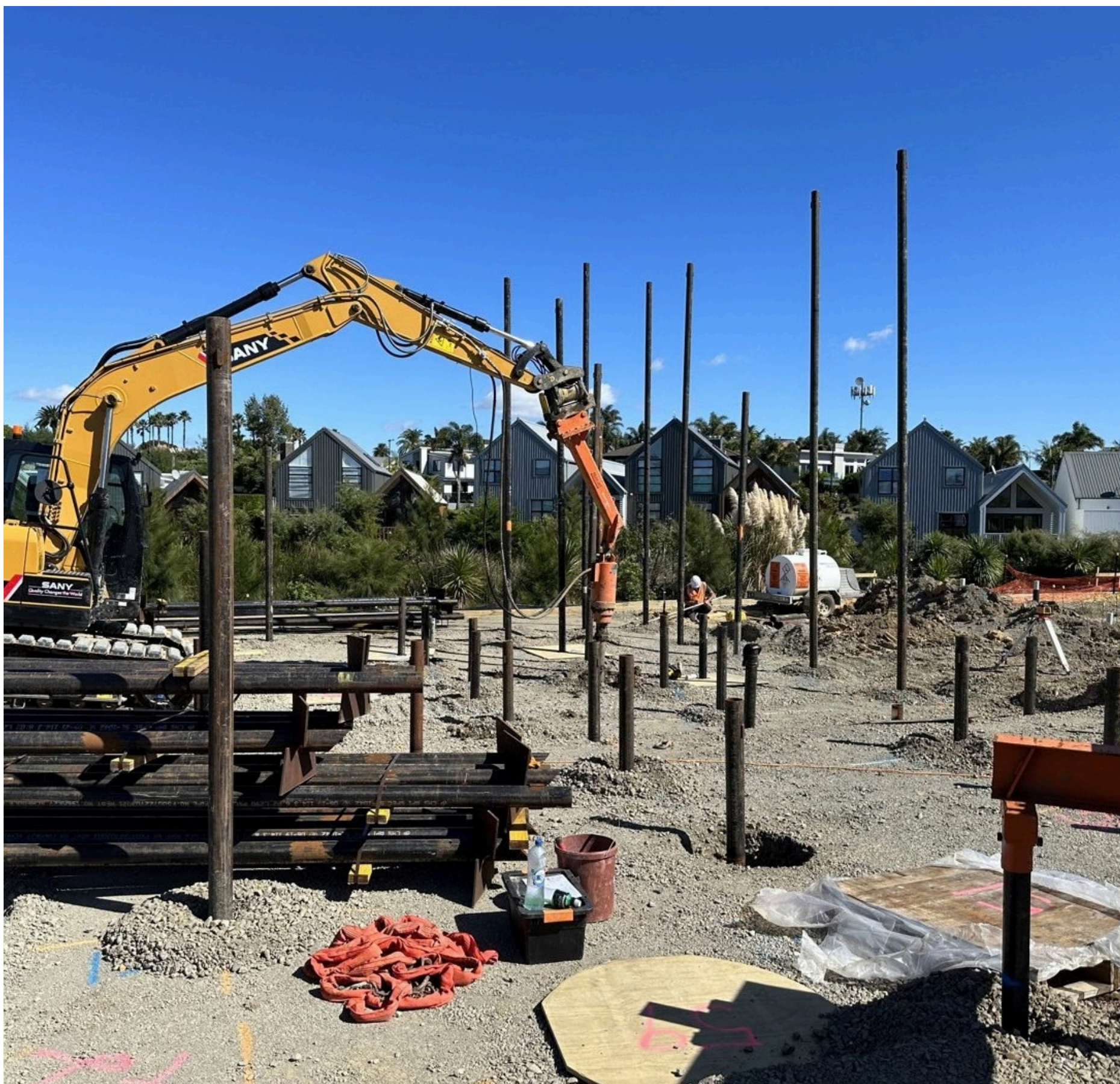
— Blade Pile installation underway.
