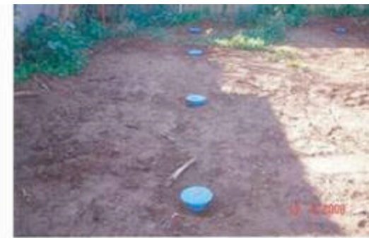
Plate C – Pile caps in place
