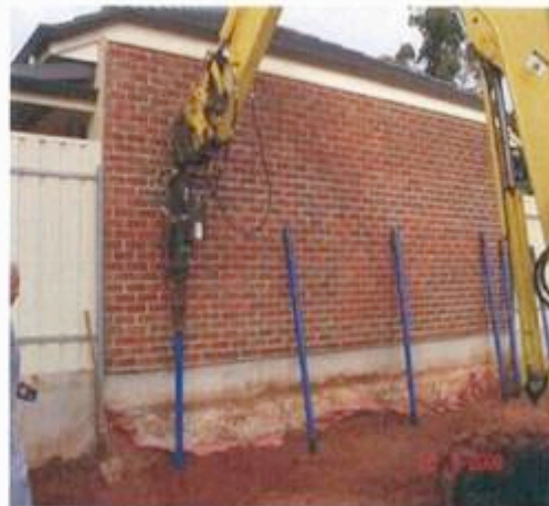
Plate B – Installation of Blade Pile
